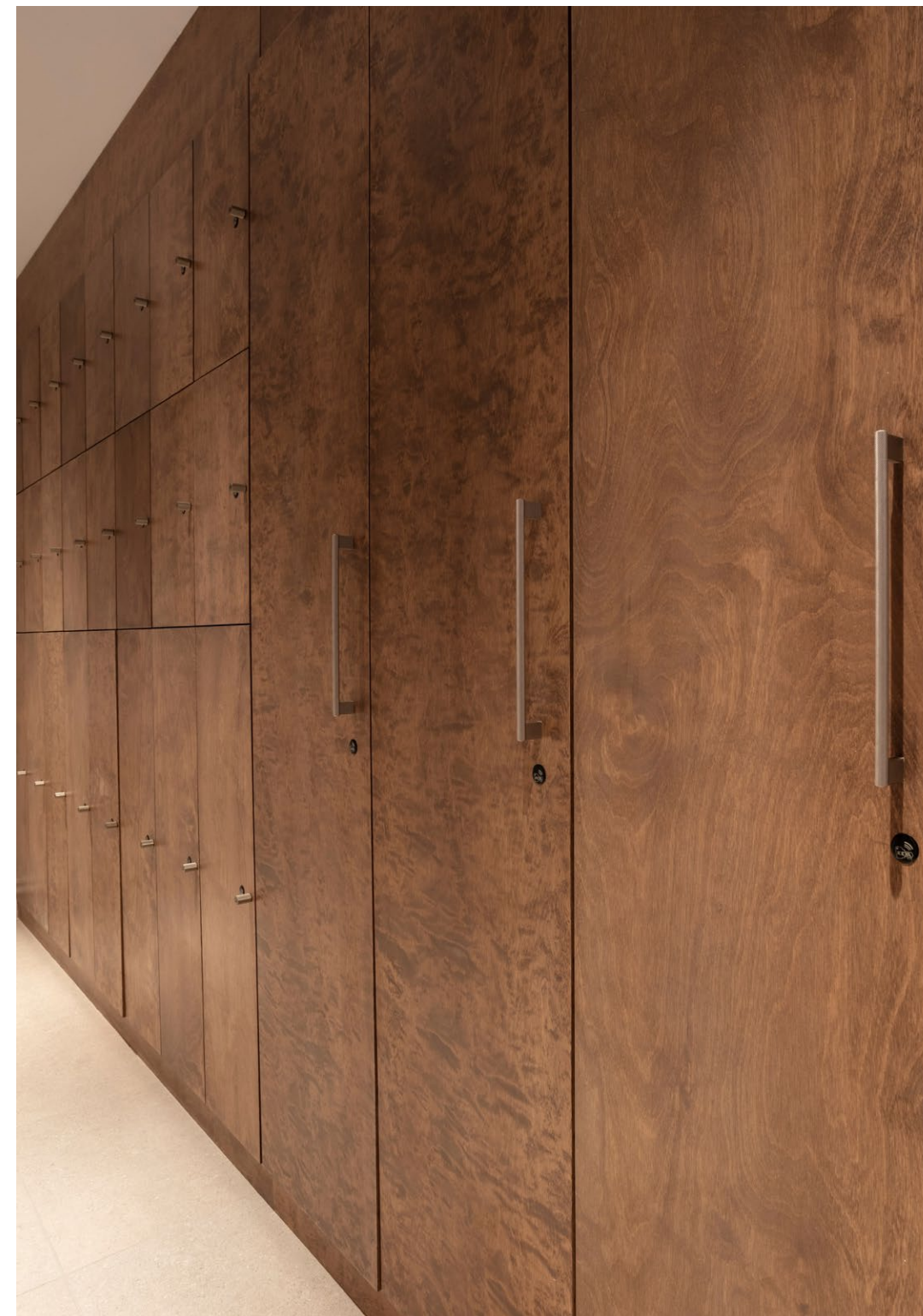
Locker Room Photograph As Built (Charlotte Square 23)
