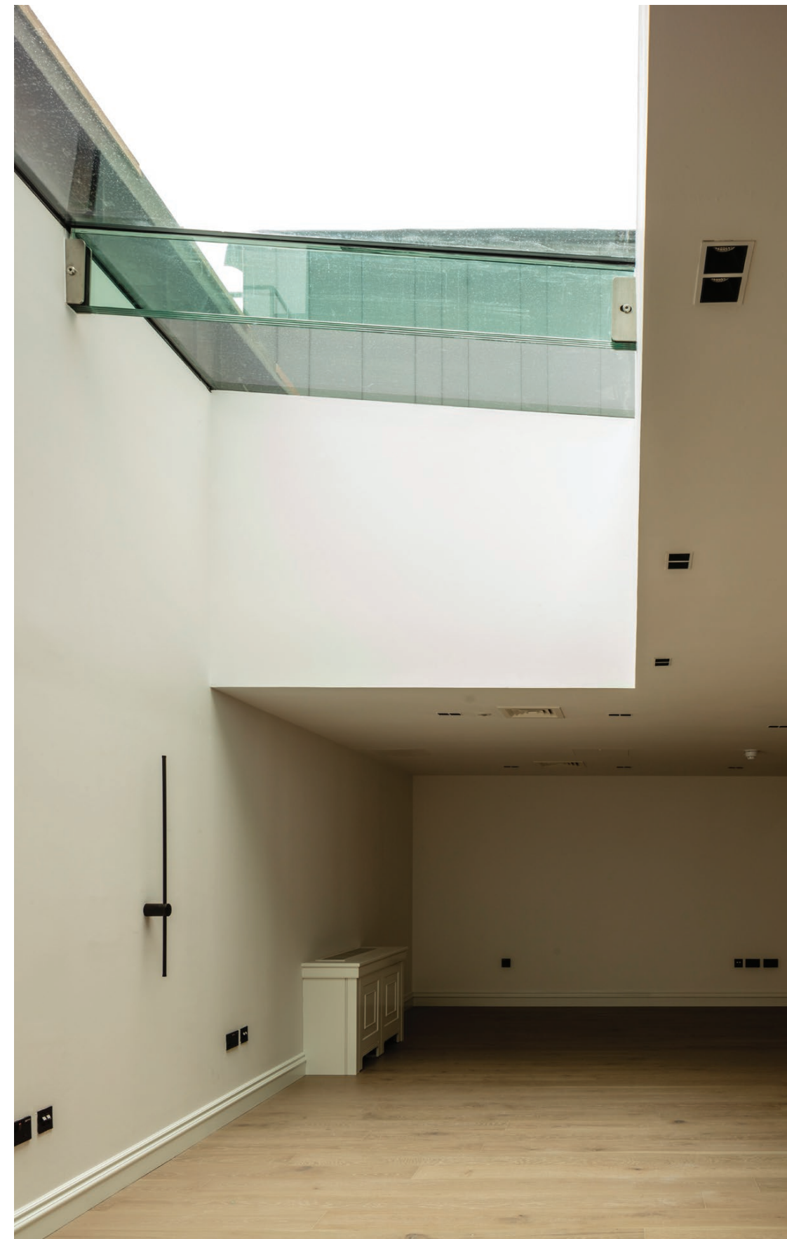
Concealed Frame Skylight Photograph as Built (Charlotte Square 22)
